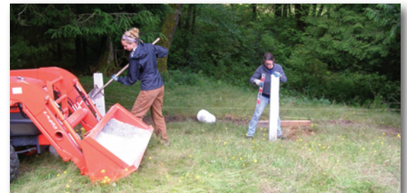
Interns Juliana Lisuk and Betsy Roberts build a fence on the Singer property to keep livestock out of Judd Creek.
